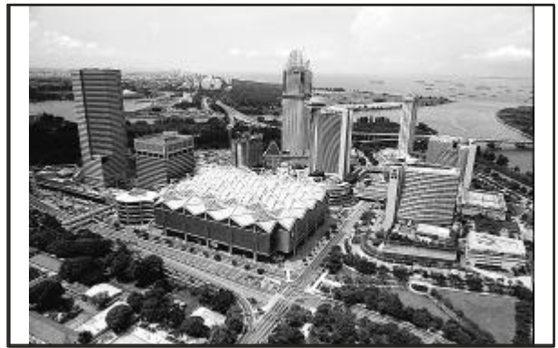
Part of Singapore skyline showing the Convention Centre where the first WTO Ministerial was held: The country's steadfast faith in the multilateral trading system was appreciated. (Photo by Steven Lee of the Straits Times)
